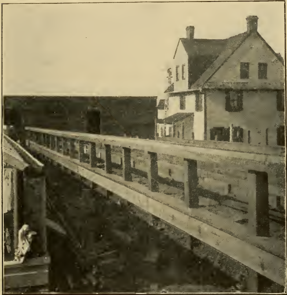
27.—Constructing house twenty-four feet wide; third step, running gutters and notching plate around posts
